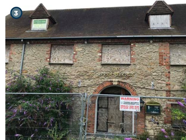
Fig 5.23: View of the vacant listed Upper Reaches building to the east of the Site
