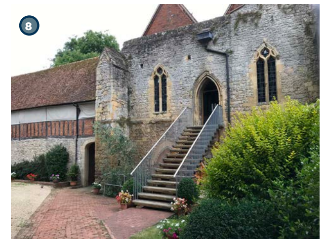
Fig 4.19: View of Abbey Checker, adjacent to the Unicorn Theatre and the Long Gallery
