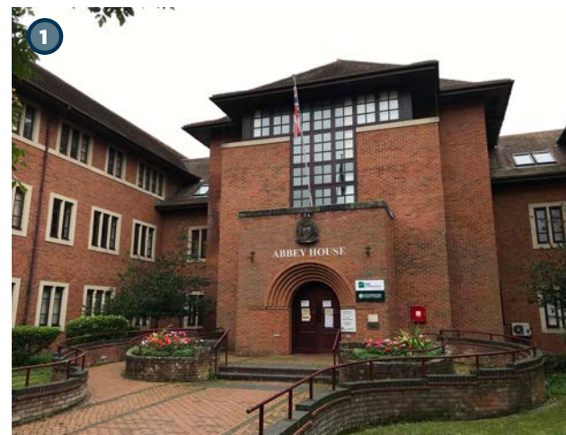
Fig 5.12: View of entrance to new Abbey House
