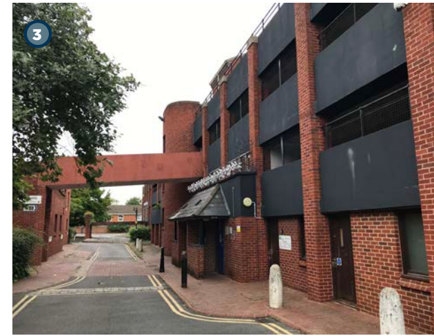
Fig 4.14: View of The Charter car park from within The Charter Site on the northern edge of the town centre
