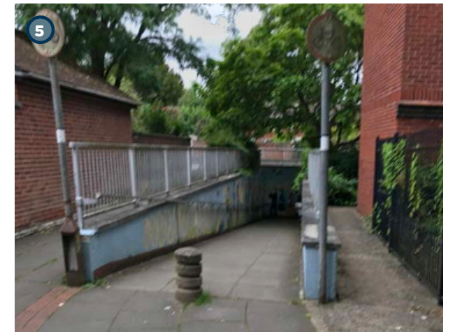
Fig 5.7: View of the pedestrian subway under Stratton Way, linking the north of Abingdon with the town centre
