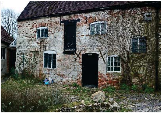
Figure 7.17: Grade II Lower Mill
