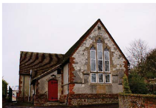
Figure 7.11: Grade II Former School, now village hall
