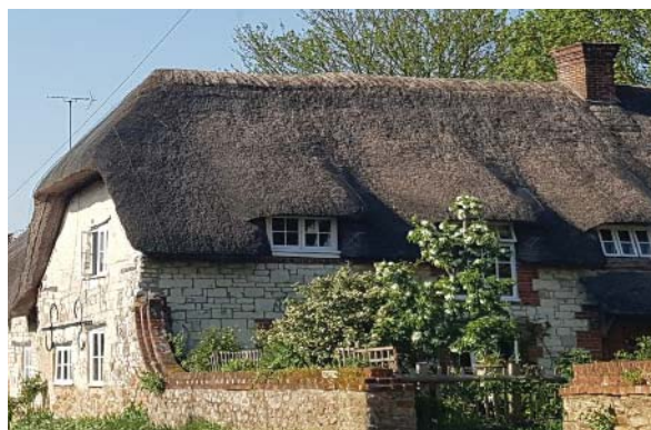
Figure 5.1: Maintaining and preserving the style of the historic buildings in the parish was of particular importance
