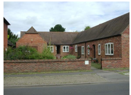
Alms Houses, High Street, Drayton
