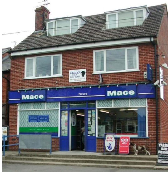
Mace Shop, Abingdon Road, Drayton
